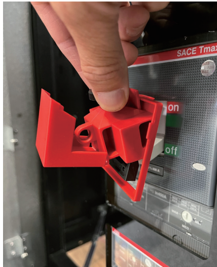
Figure 29. Remove Lock Flap
